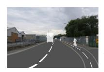
motor vehicles and pedestrian routes with new concrete kerbs. Space will be provided by narrowing the footways on both sides of the road and widening the carriageway on the eastern side of Hillam Road. The carriageway width will remain the same as at present so that access to premises can be maintained whilst also maintaining space for lorries to park.
